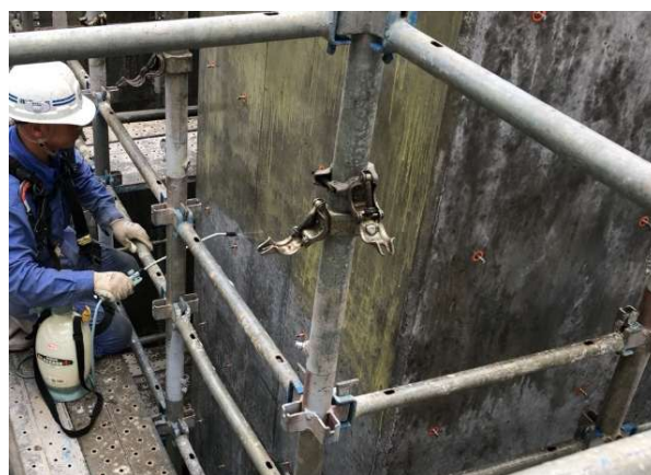
型枠取外し直後 SoyShot-20 150ml/m 2 噴霧
