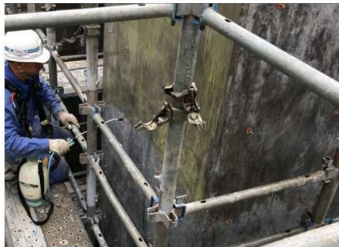
型枠取外し直後 SoyShot-20 150ml/m 2 噴霧
